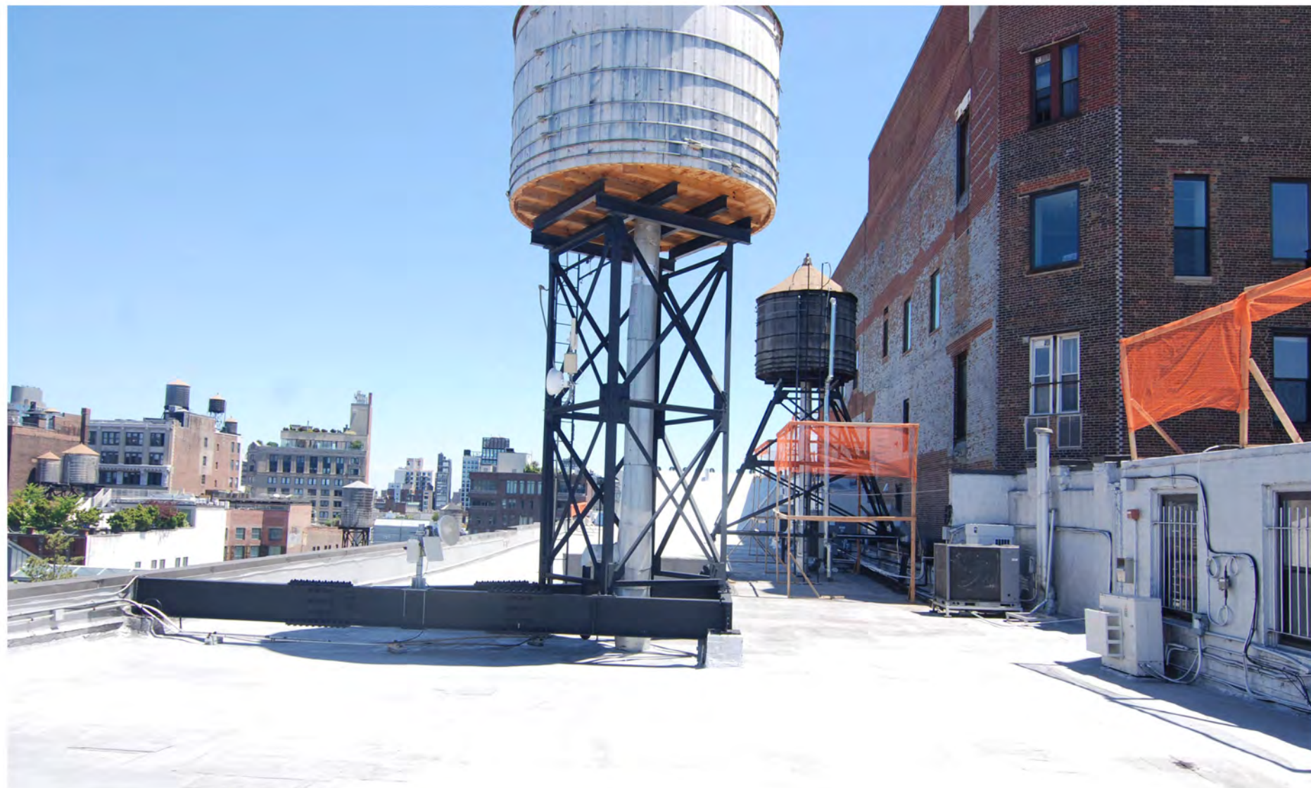
ROOFTOP MOCK UP PHOTO FACING EAST 06.17.21
