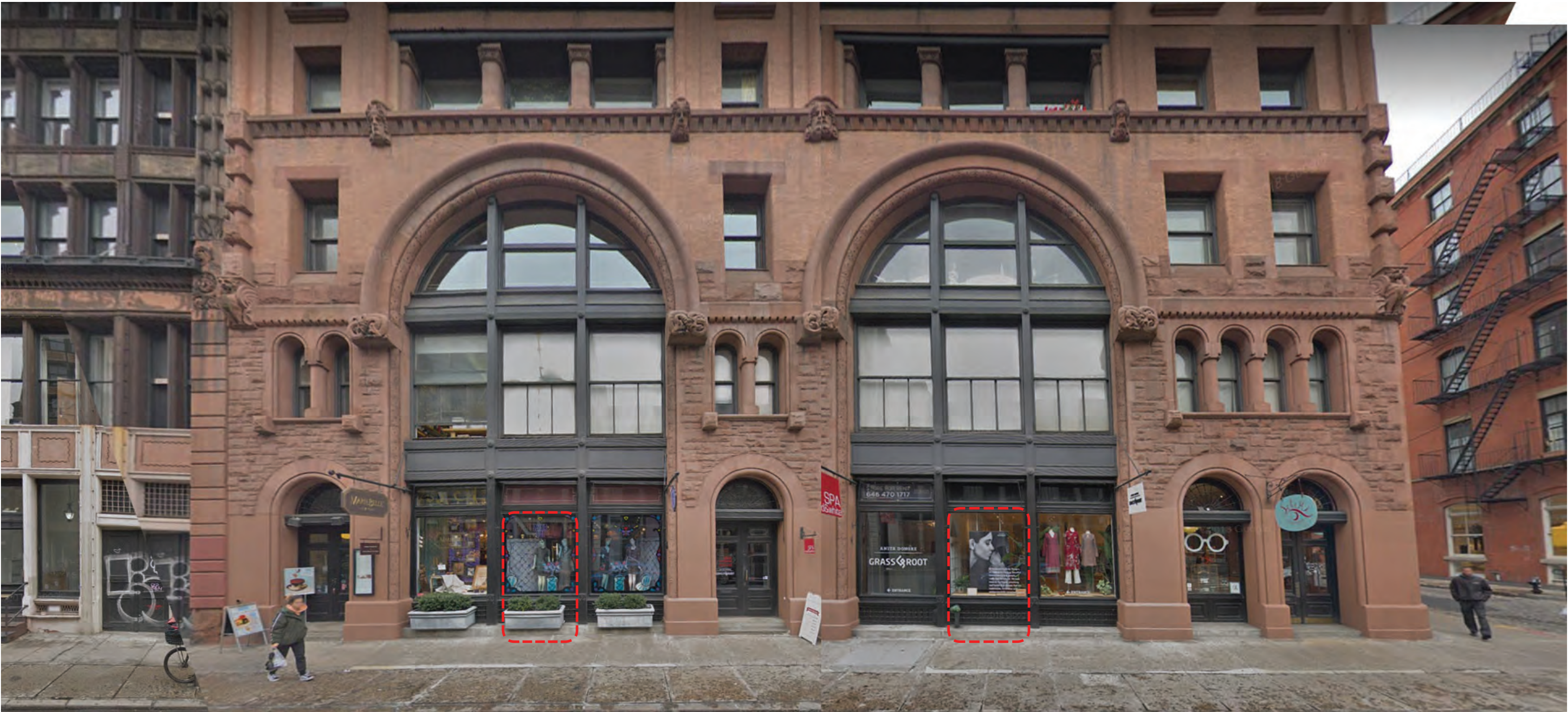
PHOTO ELEVATION OF 484 BROOME ST.
