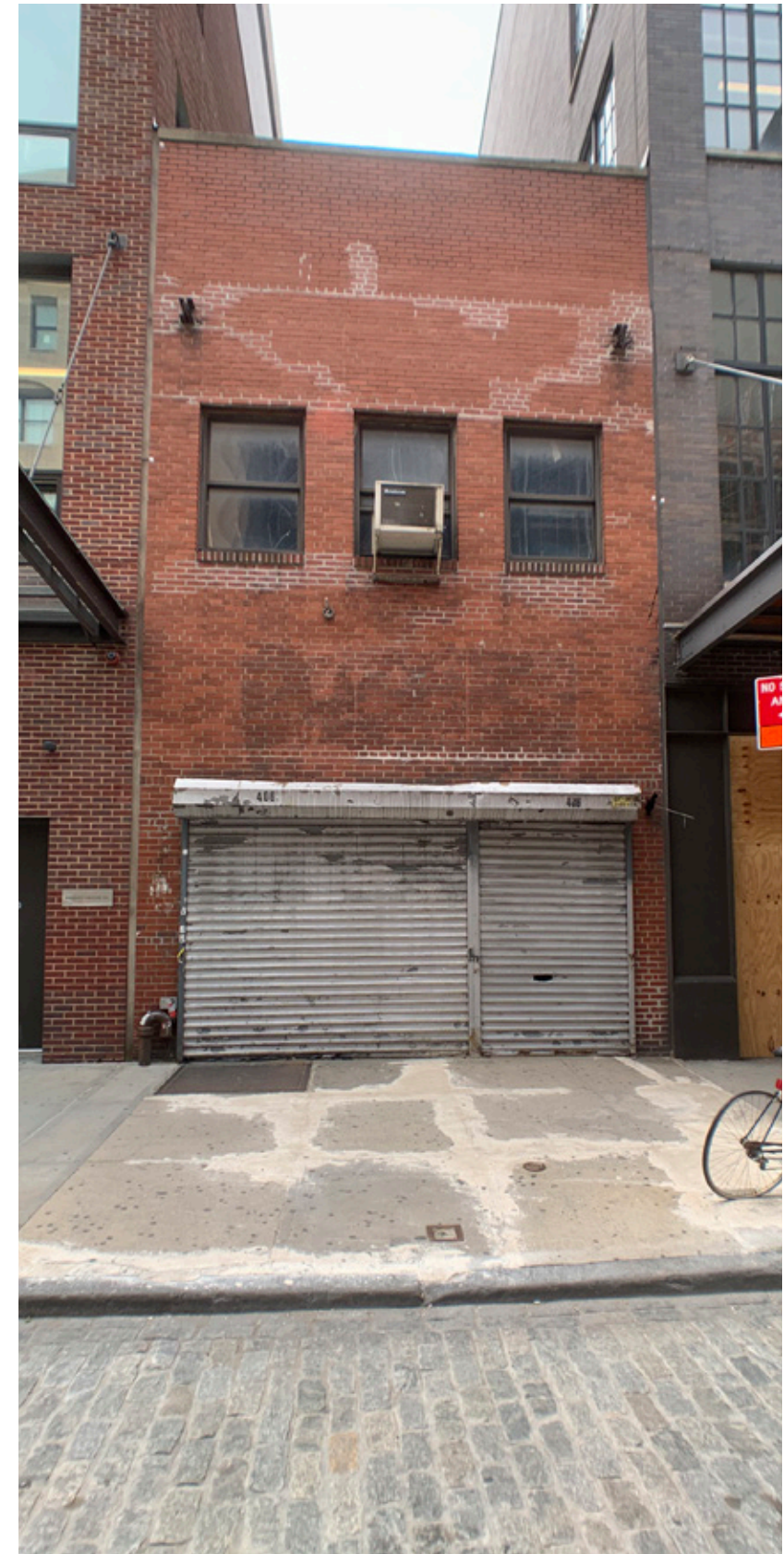
Current Condition (2021) - No Style
