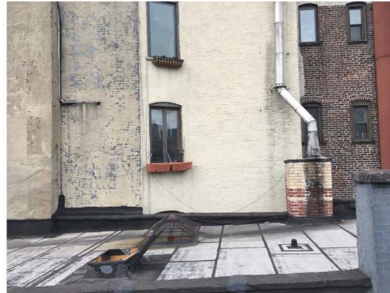
Photo #1 Looking West
