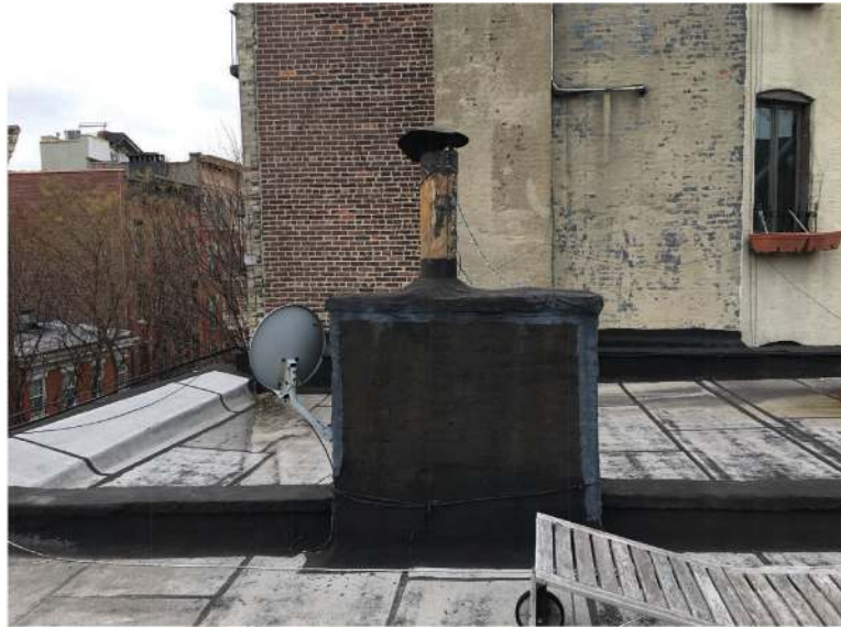
Photo #2 Looking West
