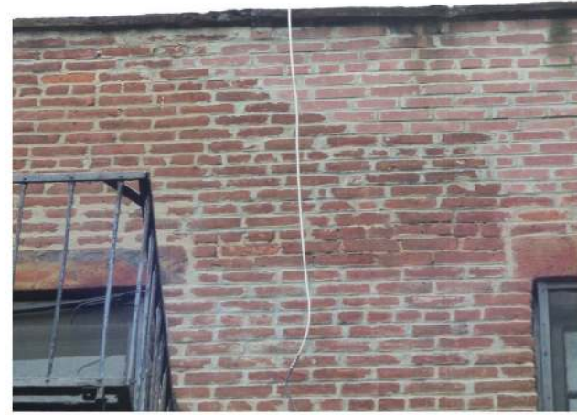
Photo # Detail Existing Conditions
