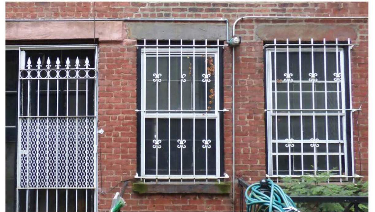
Photo #3 Detail Existing Conditions
