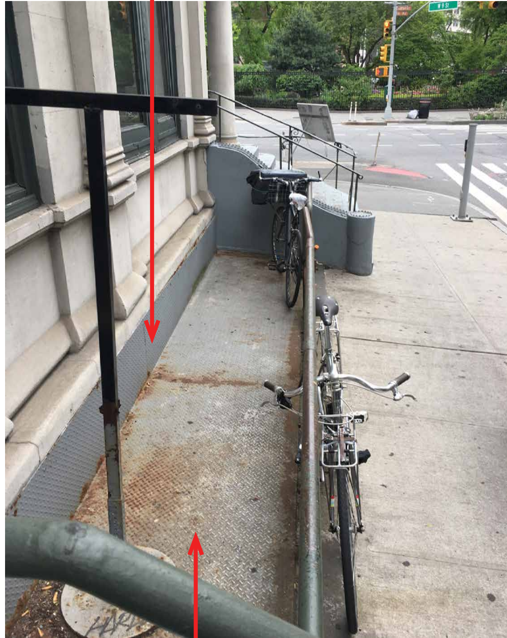
Existing Diamond Plate on Vault
