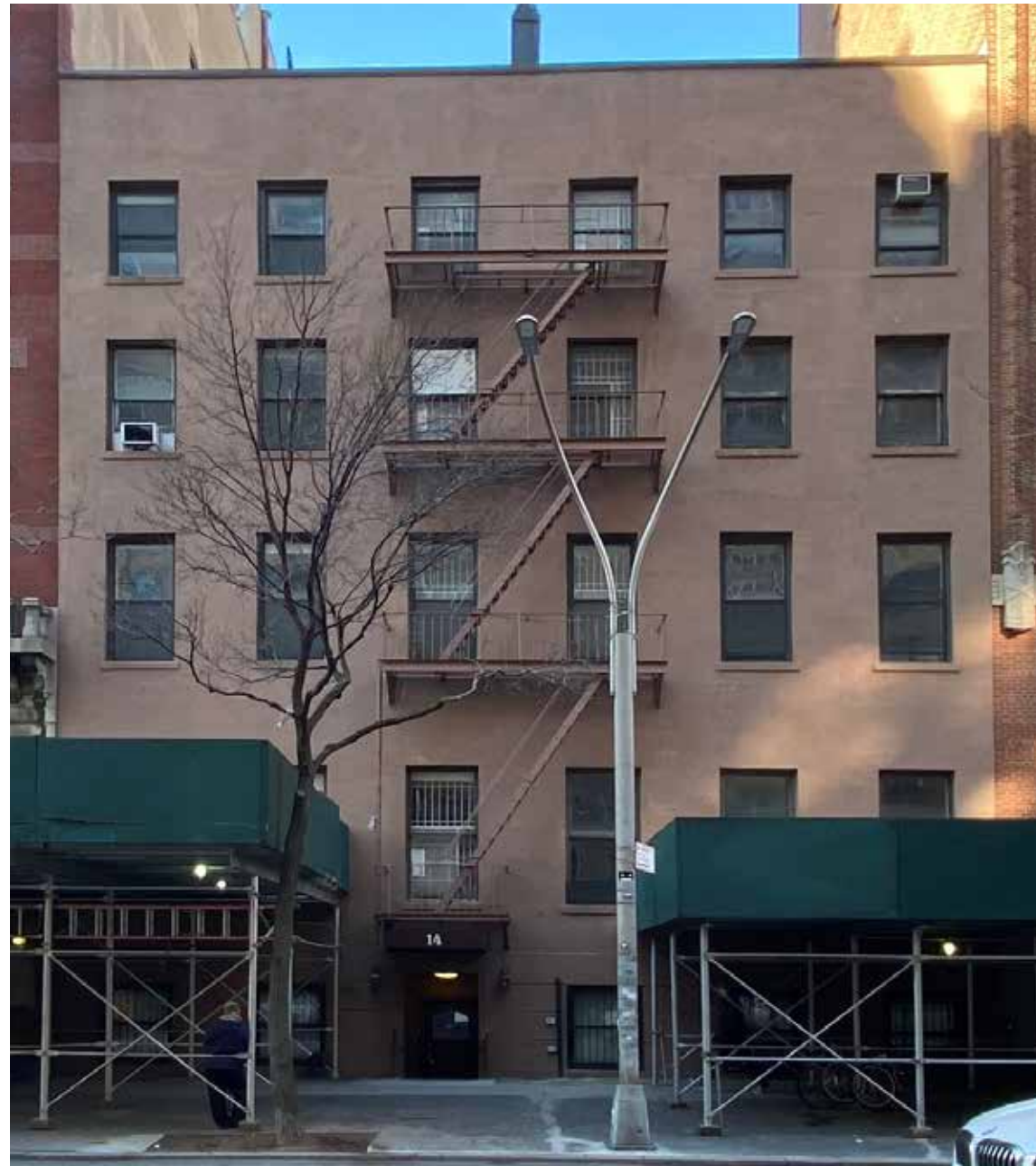
Current Building Conditions
