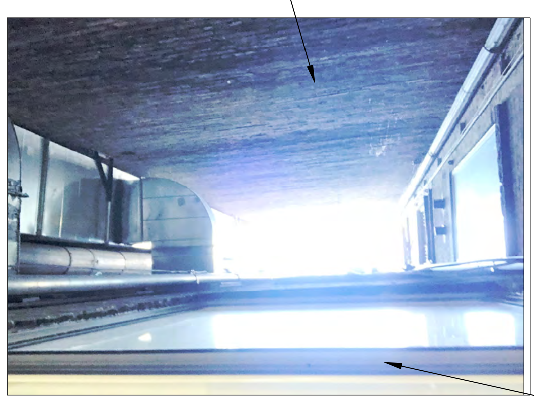
EXIST. LIGHTSHAFT @ CELLAR LEVEL LOOKING UP
