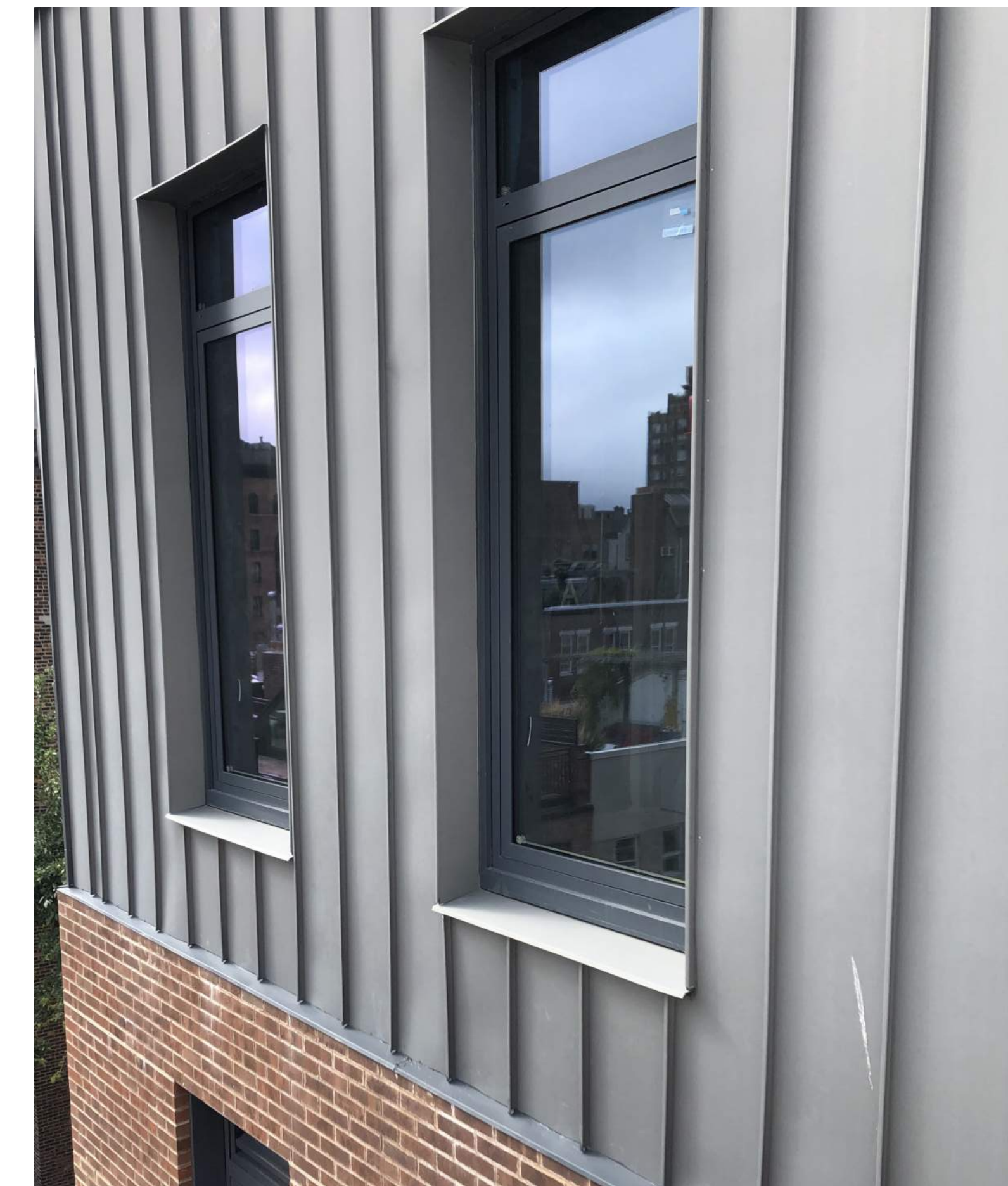
TYPICAL STANDING SEAM ZINC APPLICATION
