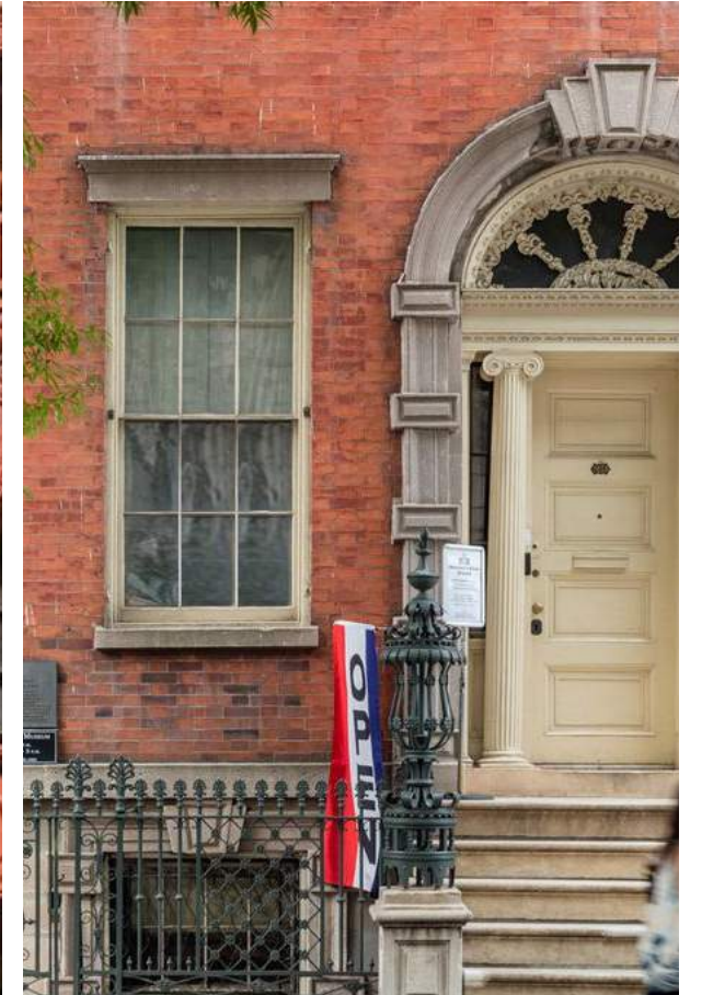
DETAIL OF BRICKWORK TONES AT THE MERCHANT'S HOUSE MUSEUM
