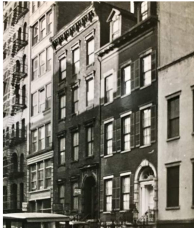
27 E 4TH STREET IN 1940S TAX PHOTO TOWNHOUSE FENESTRATION PROPORTIONS
