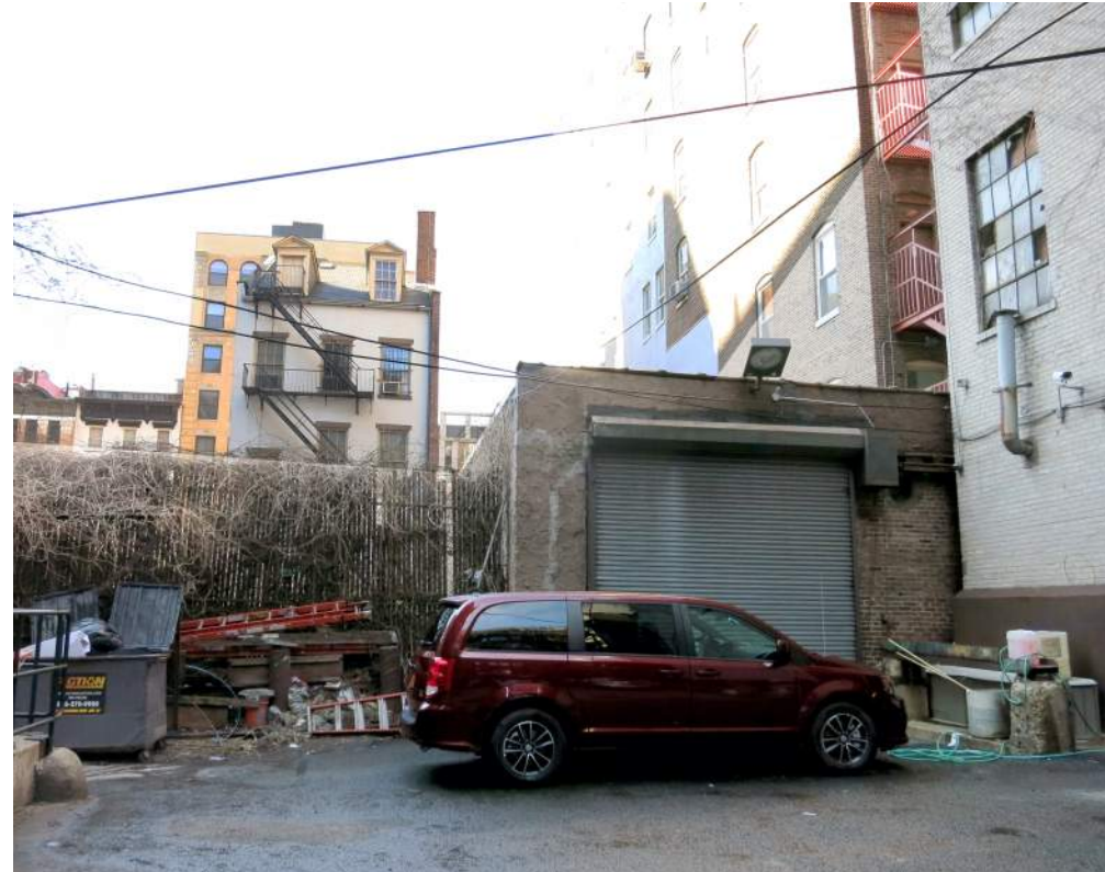
C - EXISTING CONDITIONS - STABLE COURT, FACING REAR OF LOT 72
