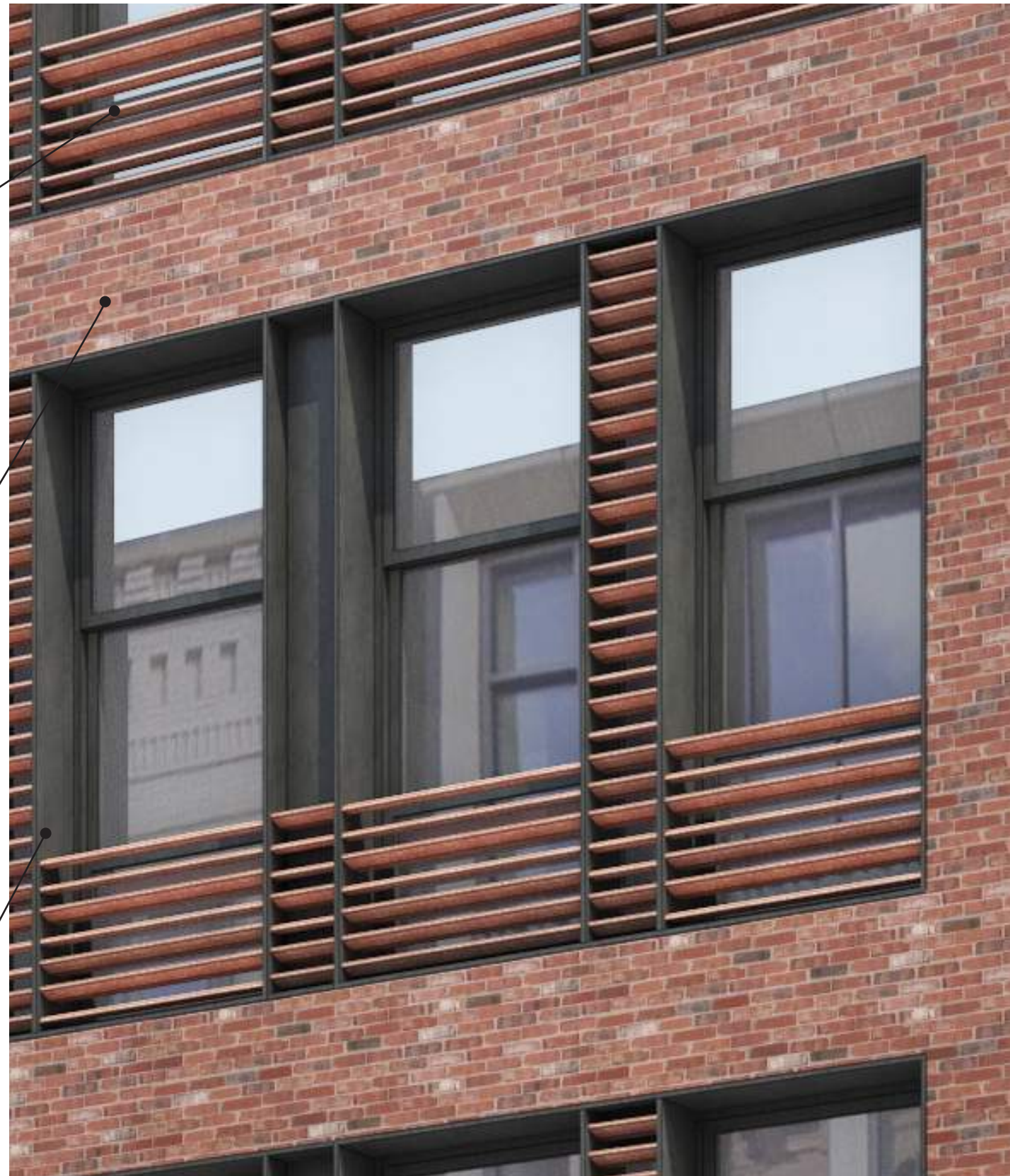
CLOSE UP OF TERRA COTTA SCREENS IN METAL FRAMES OVER CONTINUOUS WINDOWS
