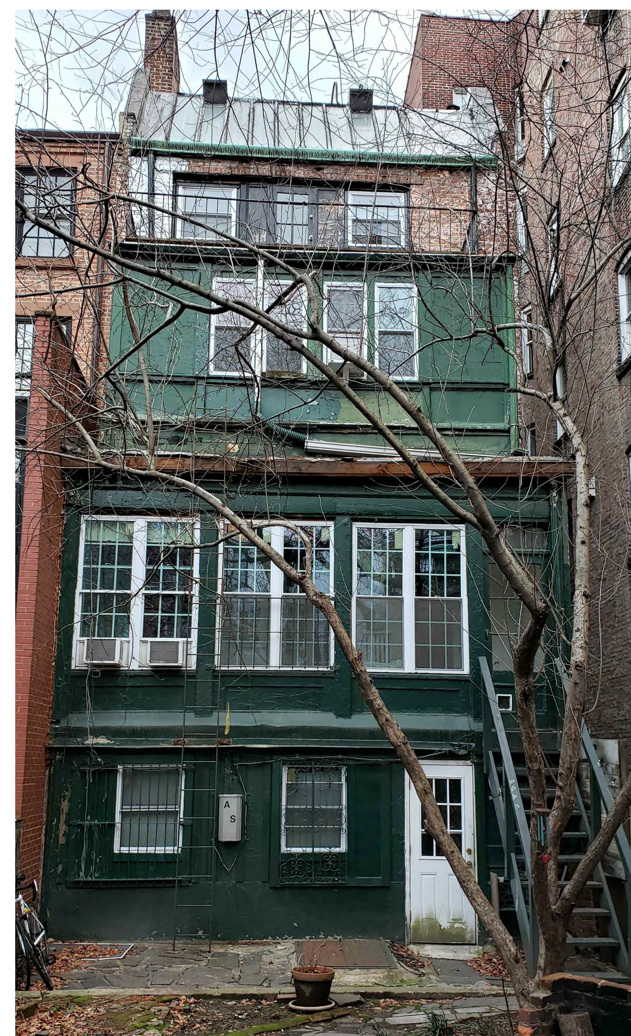
2 EXISTING PHOTO NORTH ELEVATION SCALE: 3/8"=1'-0"
