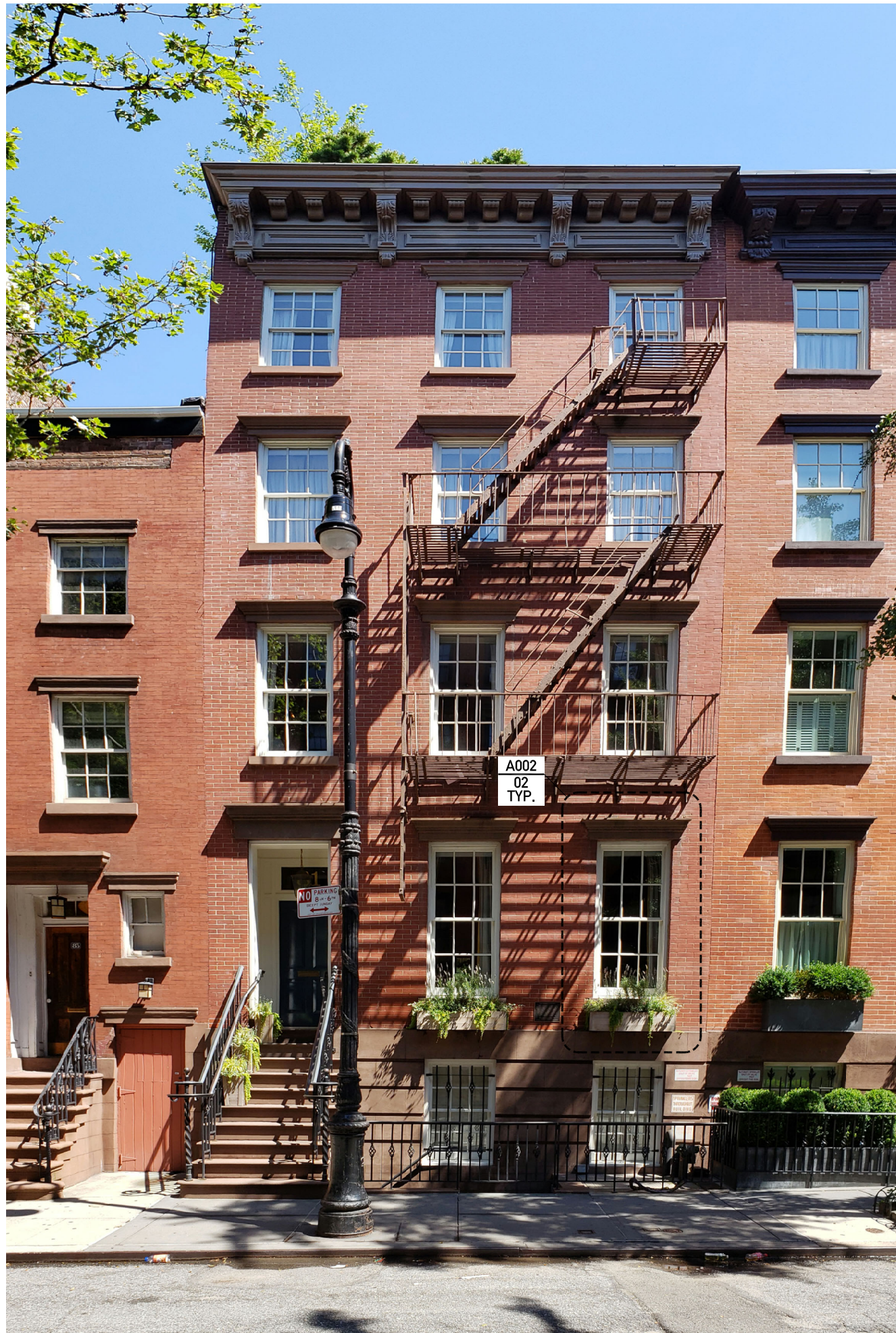
01 | EXISTING CONDITIONS PHOTO (HORATIO STREET) SCALE: N.T.S.
