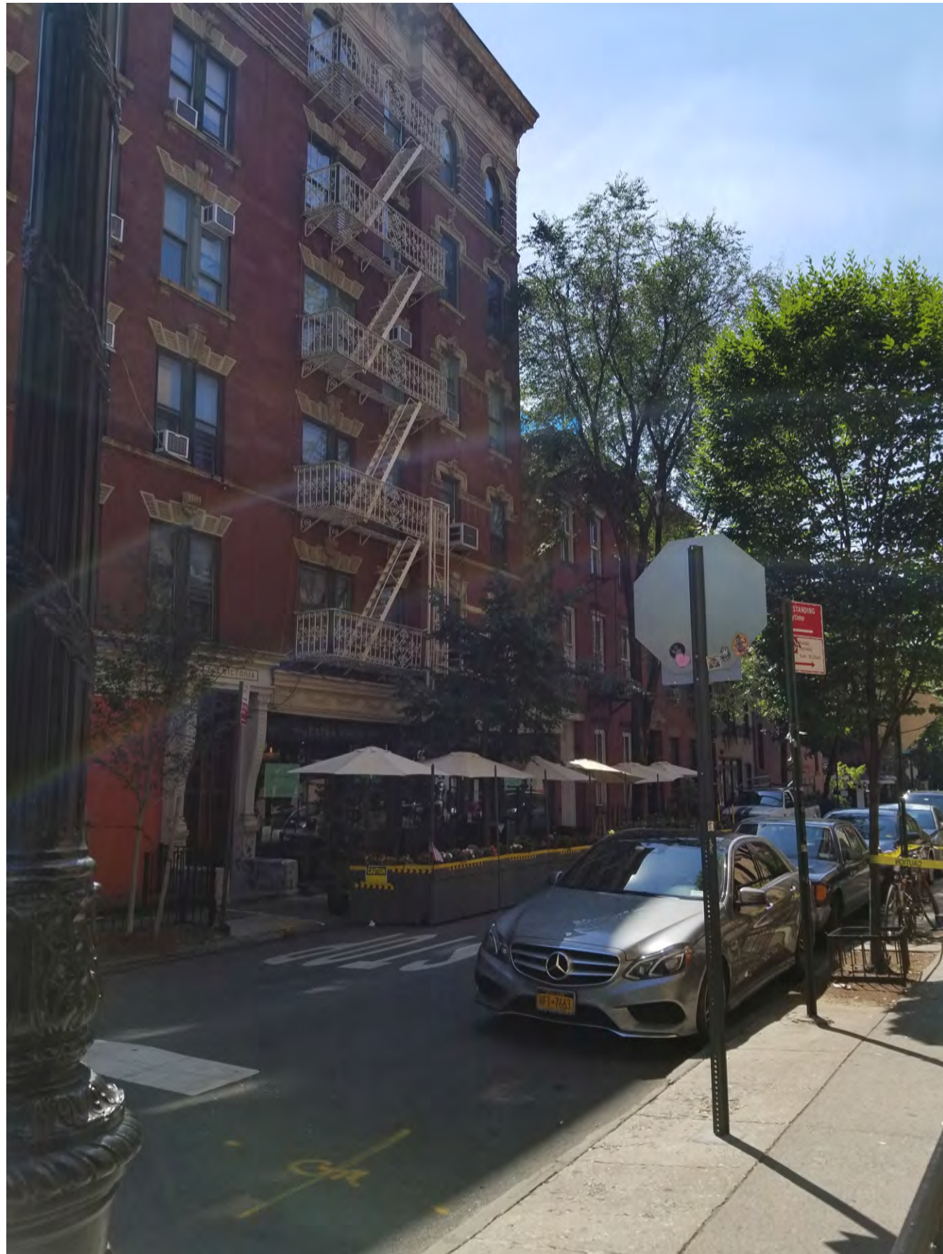
CHIMNEY & RAILING MOCKUP (VIEW FROM NORTH)
