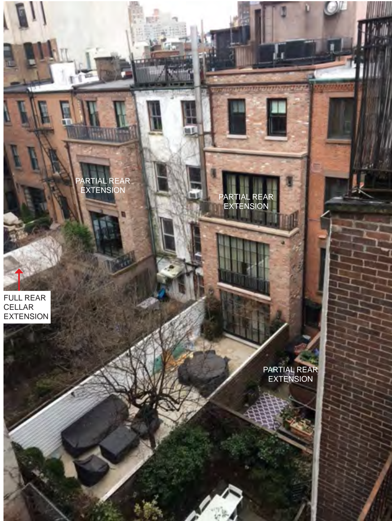
PHOTOS TAKEN FROM ROOF OF 257 WEST 4TH STREET (JANUARY)
