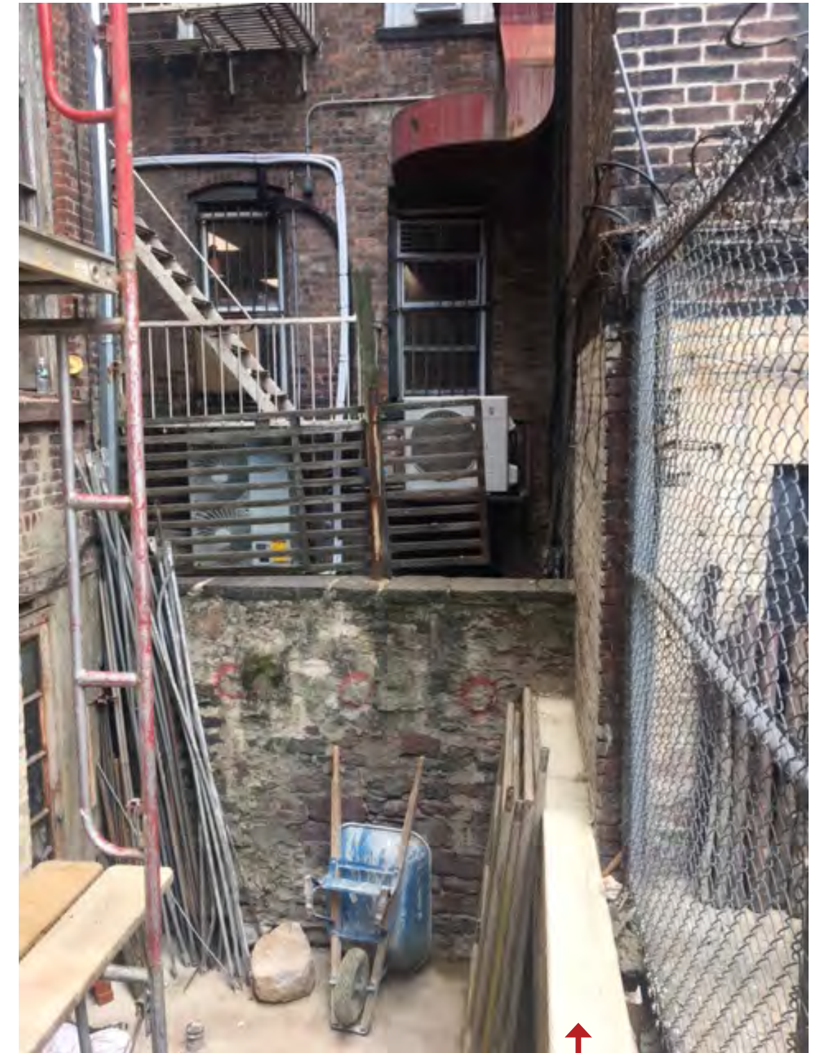
257 WEST EXISTING REAR YARD
