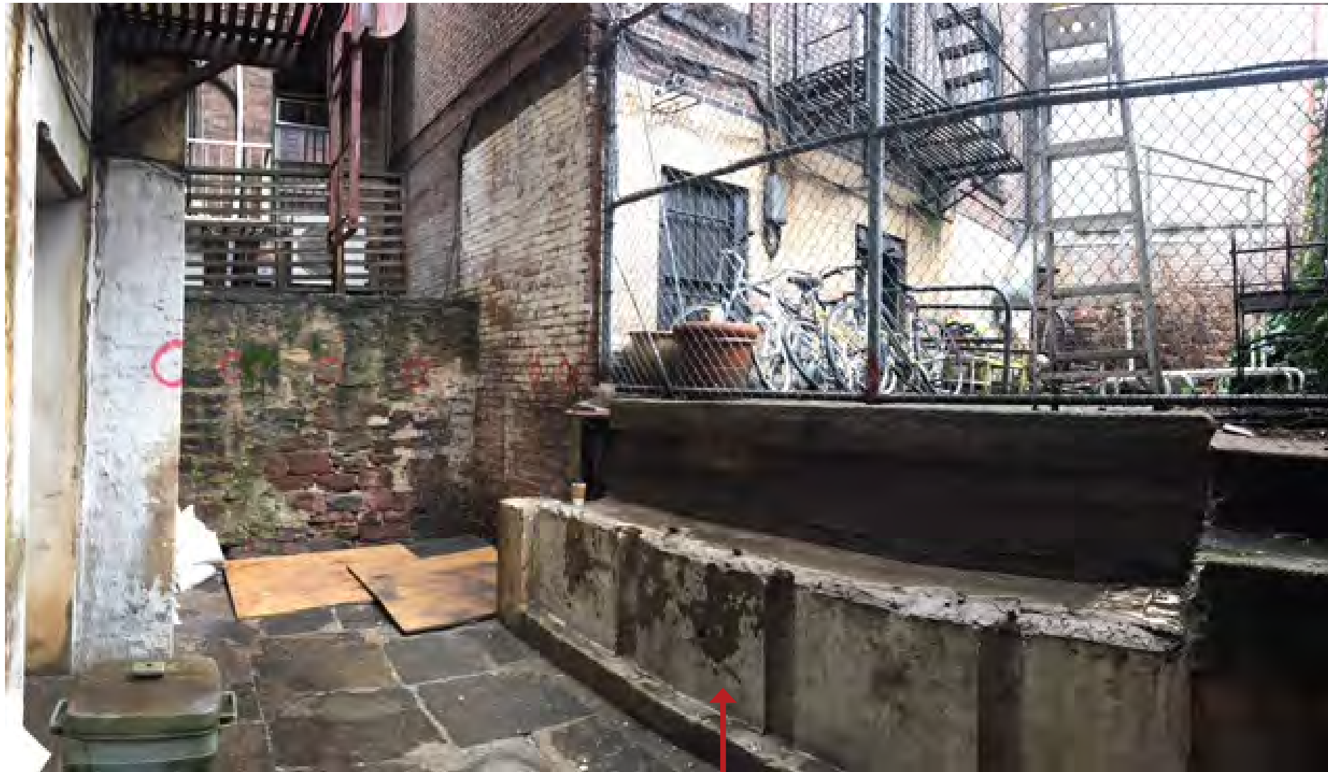
257 WEST EXISTING REAR YARD
