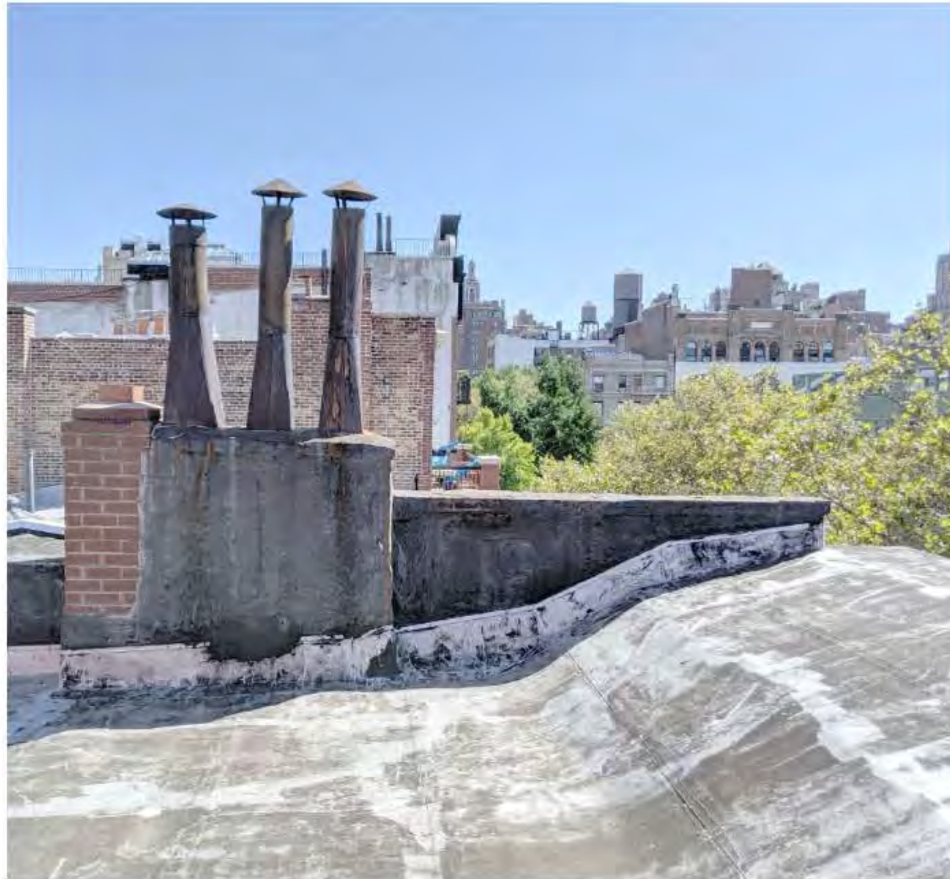
PHOTO OF FRONT CHIMNEY (DATE OF PHOTO 09/17/19) NOT TO SCALE
