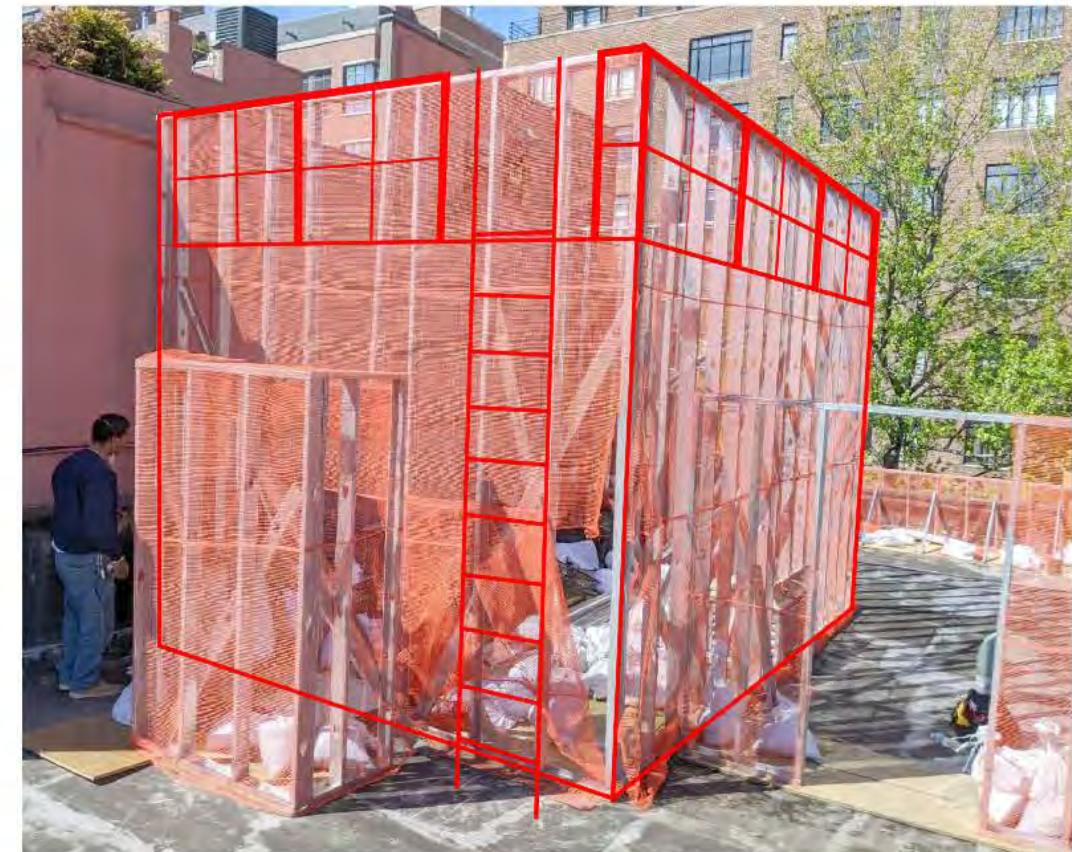
PHOTO OF ROOF MOCKUP 'D' (DATE OF PHOTO 05/12/20) NOT TO SCALE
