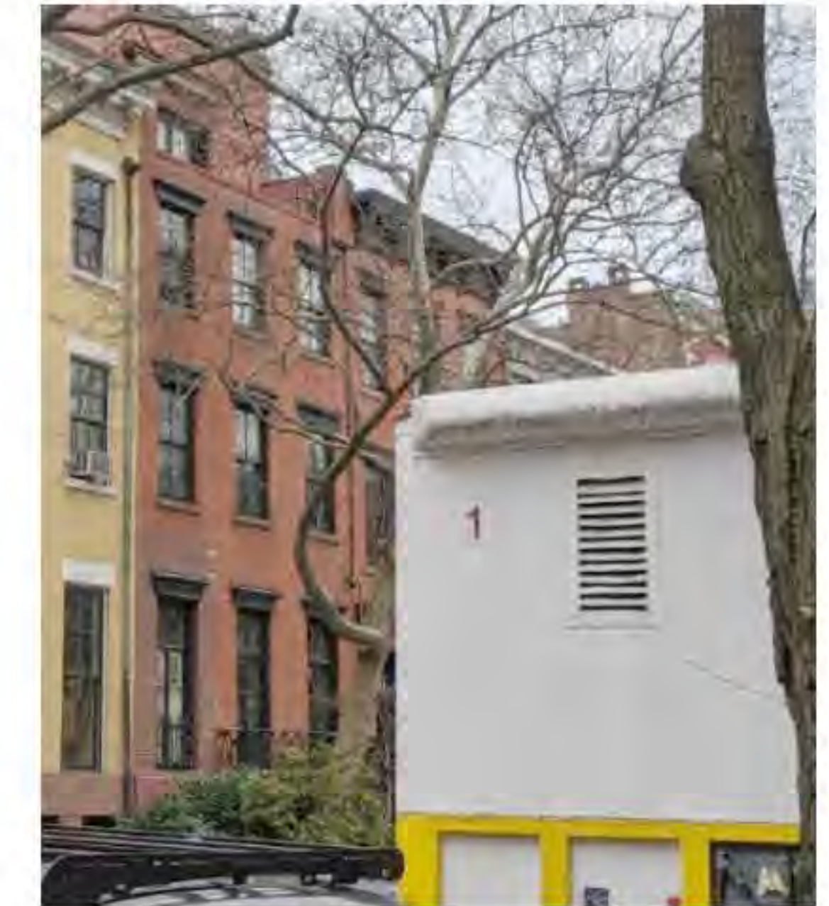
VIEW FROM SECTION 'C' (DATE OF PHOTO 03/03/20) NO SCALE
