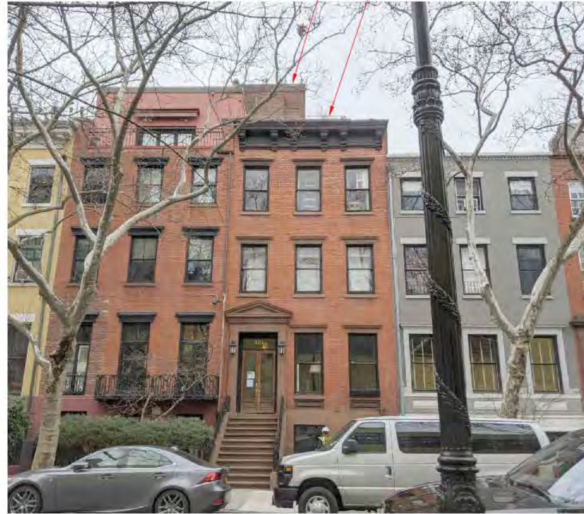
PHOTO OF ROOF MOCKUP FROM STREET 'B' (DATE OF PHOTO 03/03/20) NOT TO SCALE
