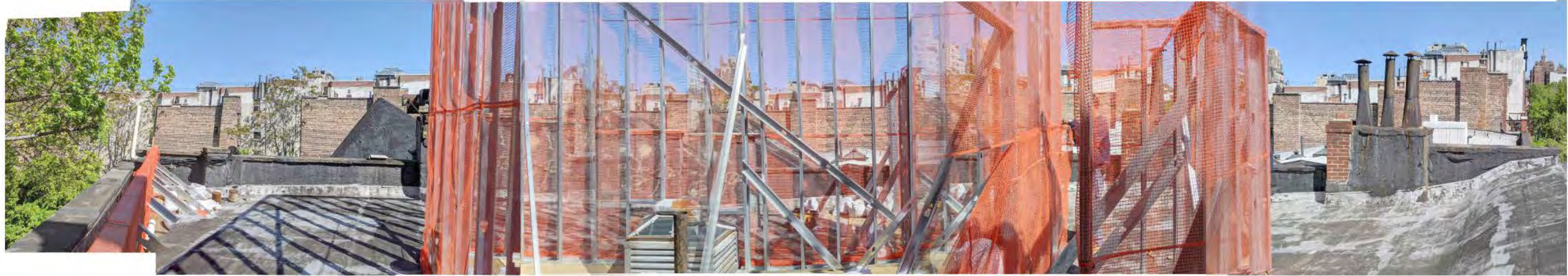
PHOTO OF ROOF MOCKUP FACING #119 (DATE OF PHOTO 05/12/20) NOT TO SCALE
