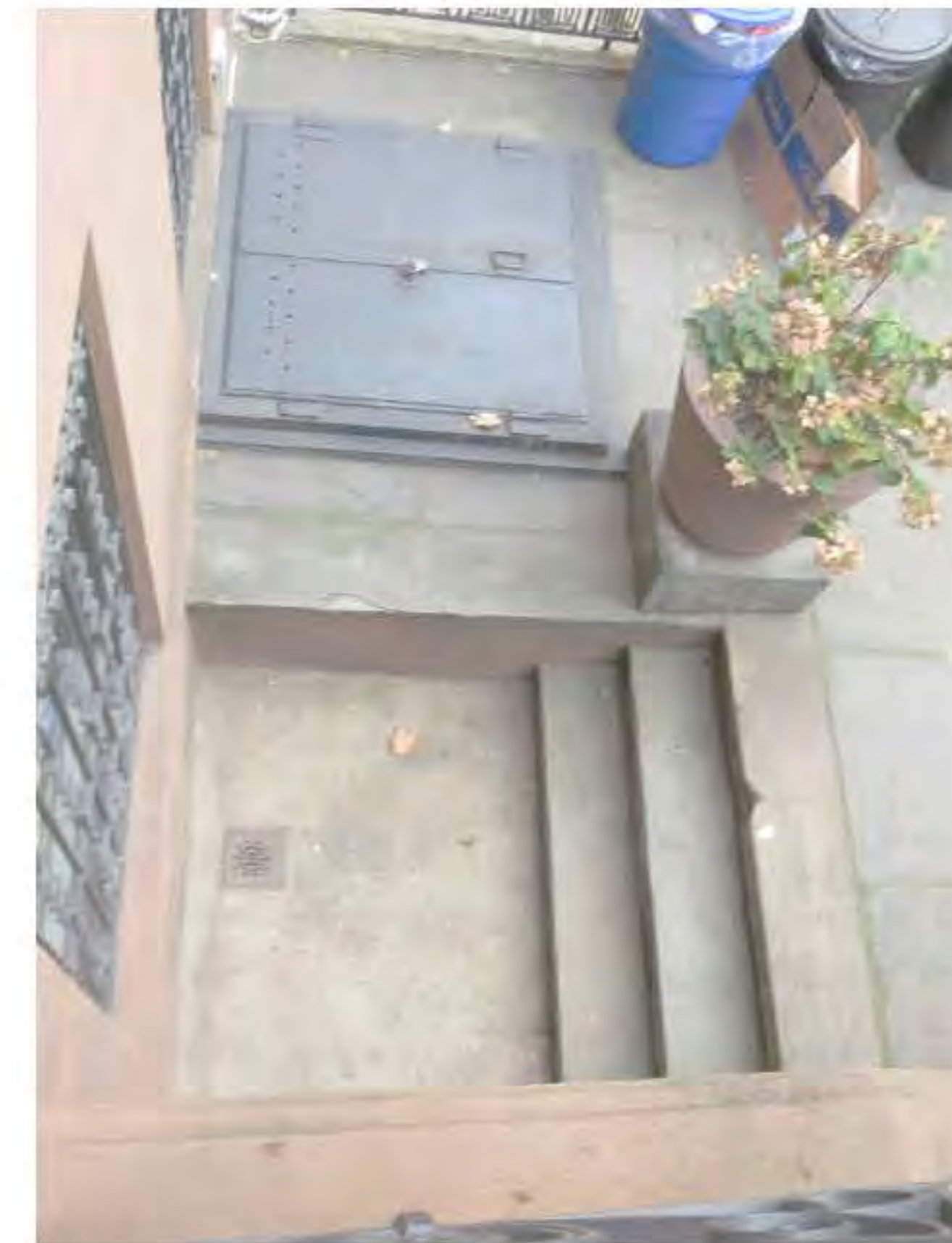
PHOTO OF LANDING AT AREAWAY (DATE OF PHOTO 09/17/19) NOT TO SCALE
