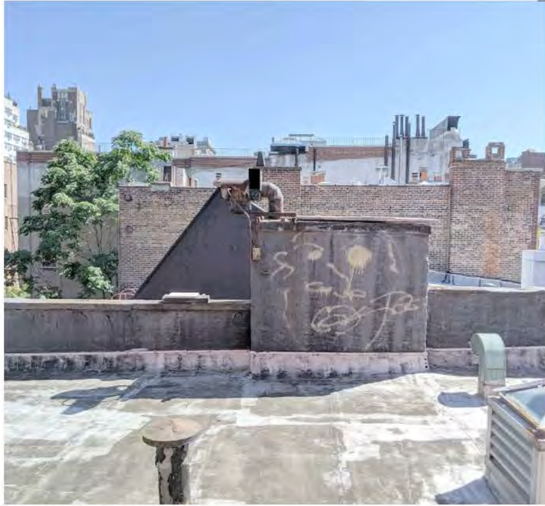
PHOTO OF REAR CHIMNEY (DATE OF PHOTO 09/17/19) NOT TO SCALE
