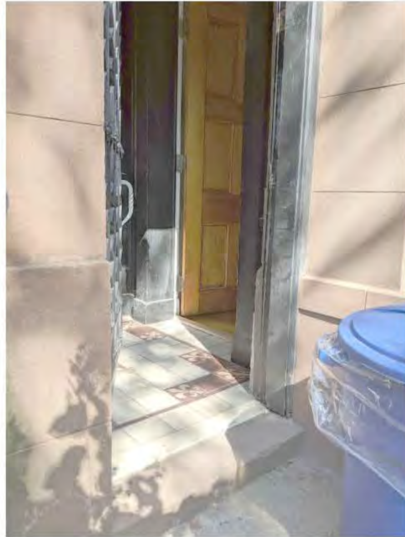
PHOTO OF VESTIBULE FROM AREAWAY (DATE OF PHOTO 09/17/19) NOT TO SCALE
