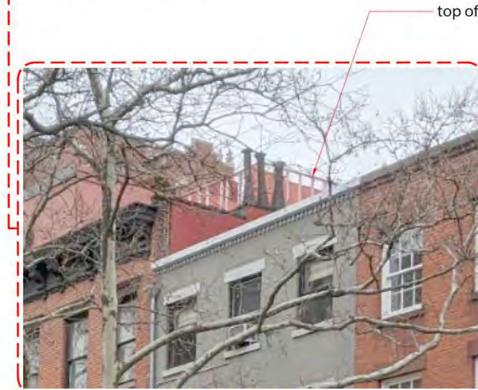
CLOSEUP PHOTO OF ROOF MOCKUP FROM STREET 'C' (DATE OF PHOTO 03/03/20) NOT TO SCALE
