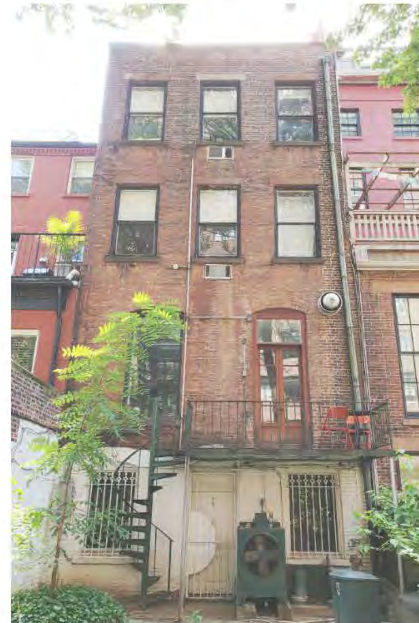
EXISTING REAR FACADE (DATE OF PHOTO 06/28/19) NOT TO SCALE
