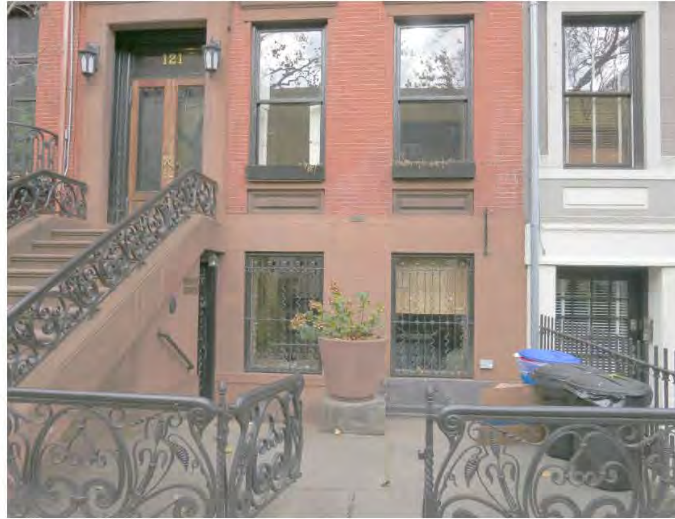
PHOTO OF FRONT YARD AREA (DATE OF PHOTO 06/28/19) NOT TO SCALE
