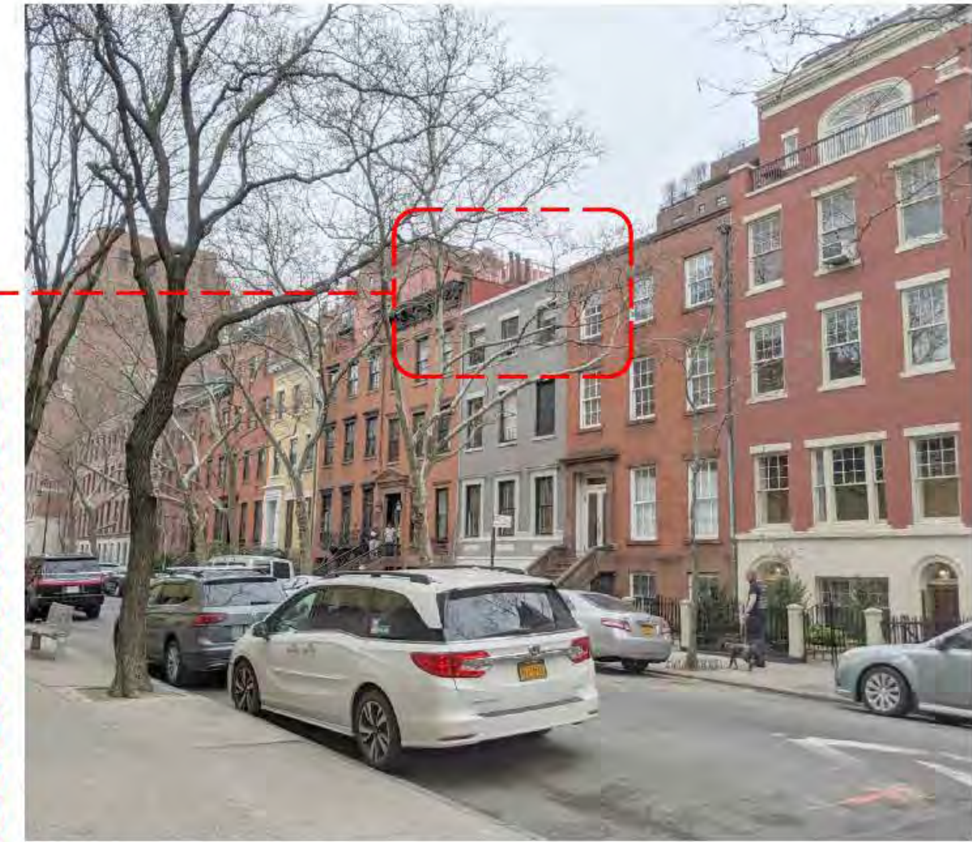
PHOTO OF ROOF MOCKUP FROM STREET 'C' (DATE OF PHOTO 03/03/20) NOT TO SCALE
