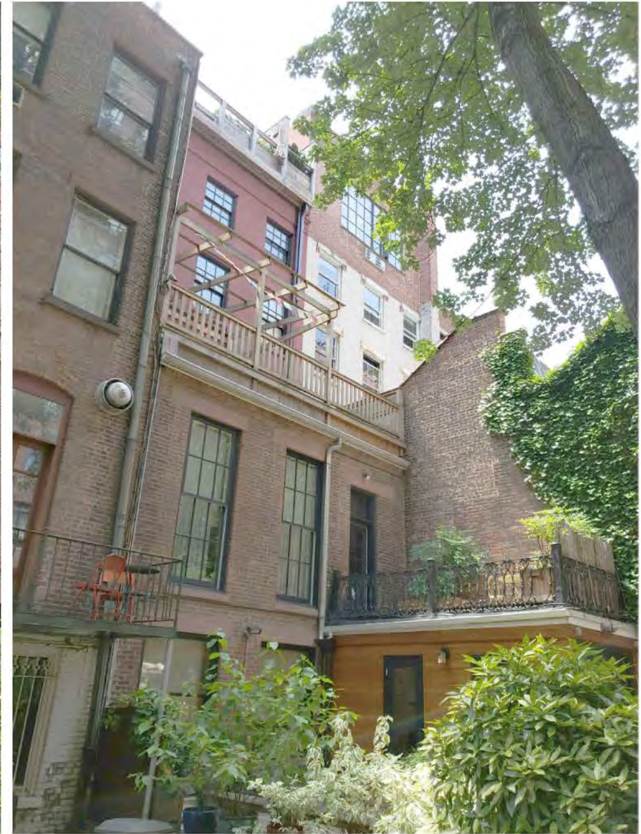
PHOTO OF REAR FACADE - 123 W 11TH ST (DATE OF PHOTO 07/22/19) NOT TO SCALE
