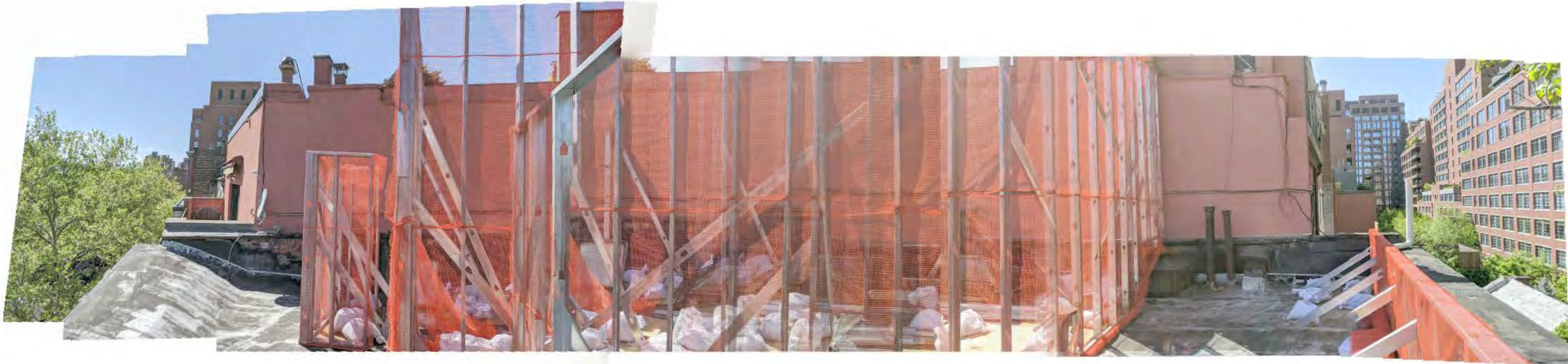
PHOTO OF ROOF MOCKUP FACING #123 (DATE OF PHOTO 05/12/20) NOT TO SCALE
