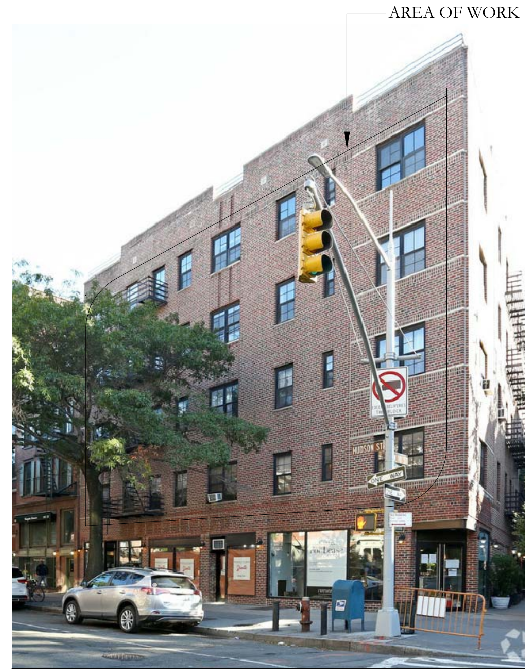
BUILDING FACADE @ HUDSON STREET
