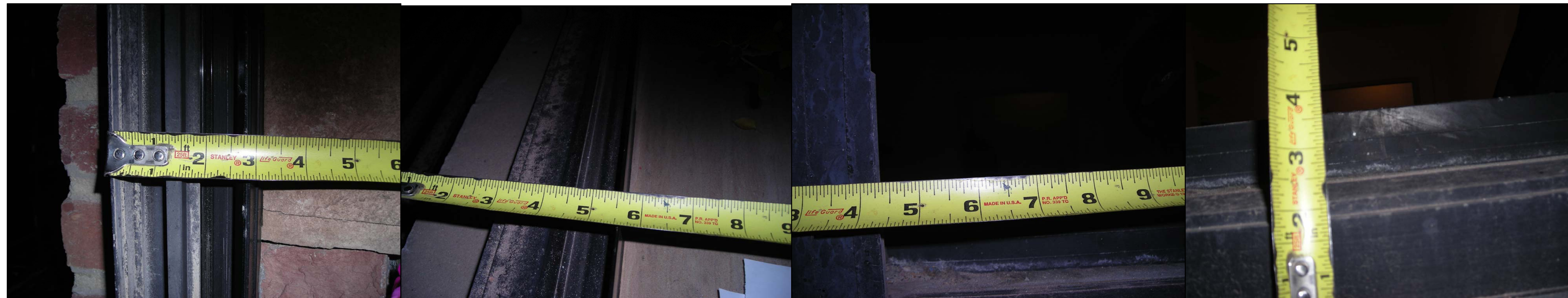
EXTG. MULLION AND BRICKMOLD
