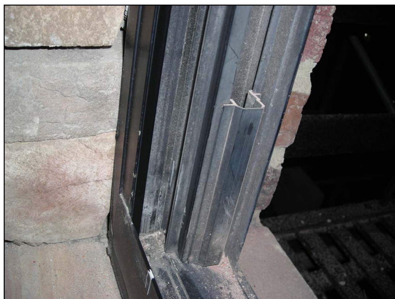
EXTG. MULLION AND BRICKMOLD
