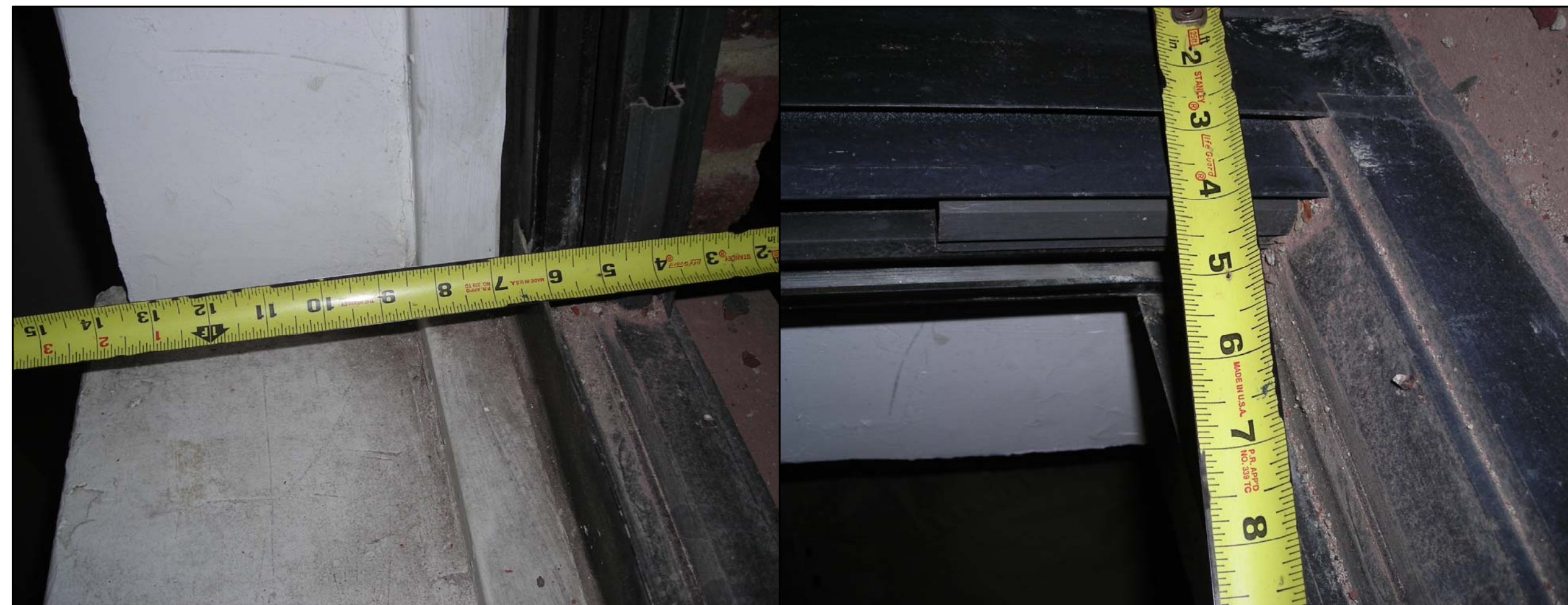
EXTG. MULLION AND BRICKMOLD
