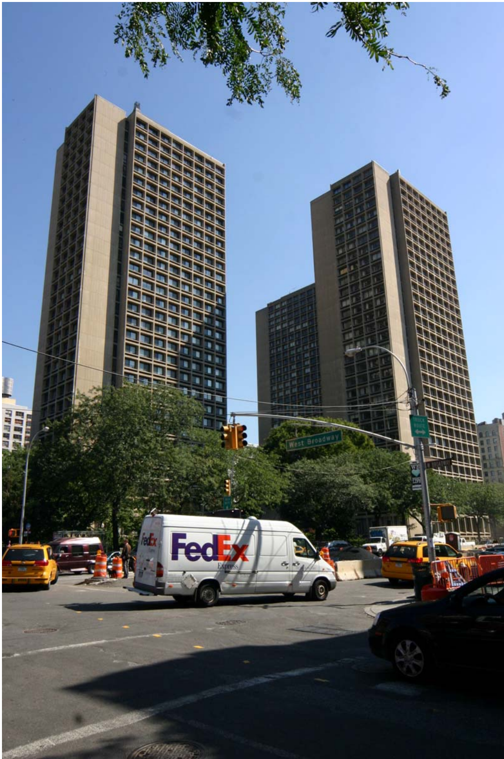
View northeast from corner of West Houston Street and West Broadway
