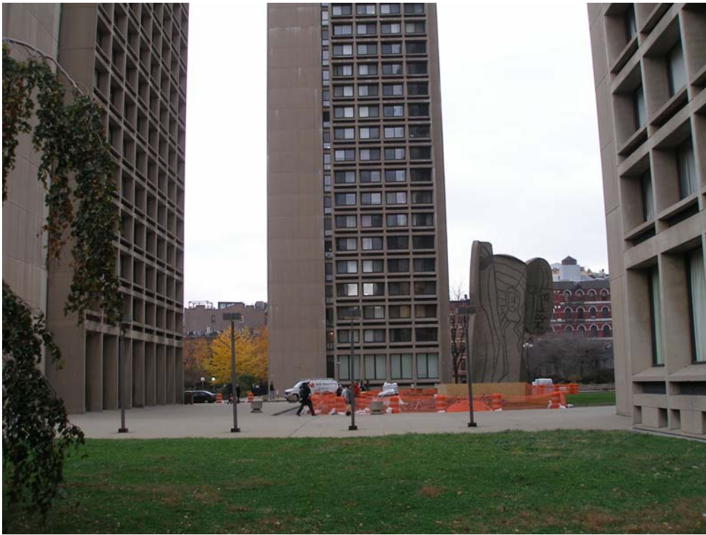
View west toward central lawn, 505 LaGuardia Place at center
