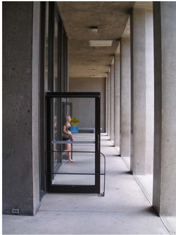
Arcade, 100 Bleecker Street, view south
